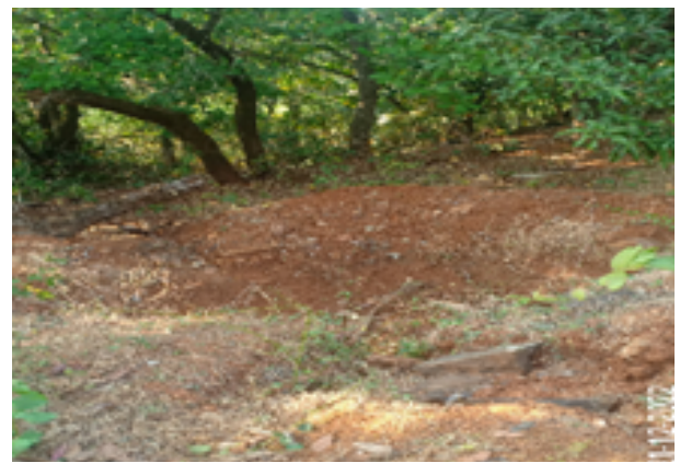
Excavation of public drains and manure pits at Mauje Kunkavan
