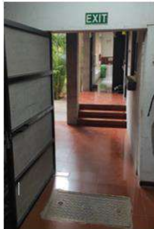
Directional exit signages
