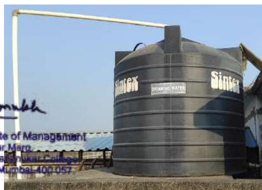
Water tank available
